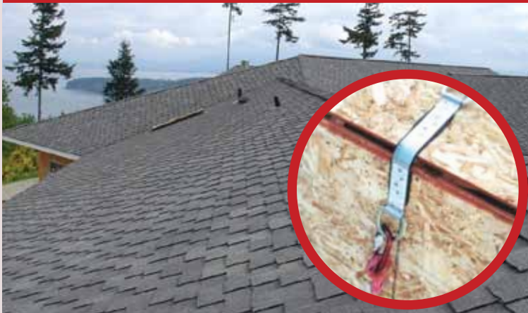
Attach D-ring to Rafter
