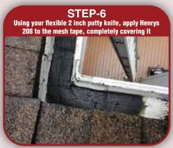
You have now repaired the leak at your gutter seams. This method is a long-lasting, quick way to patch leaky gutters. The asphalt covers the leak and the mesh tape stops the asphalt from splitting in hot or cold weather. Although this was not our invention, we have used it with great success, and we hope it works for you too!
